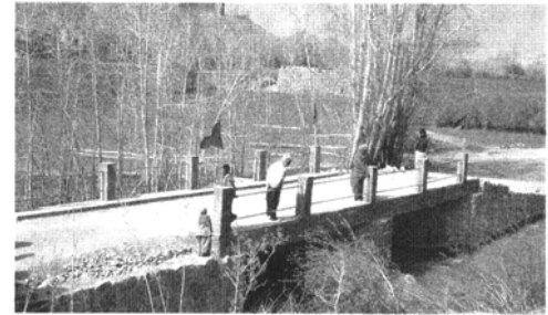
Brückenbau des ARC in Pul-e-Haji, Malistan, 1991
